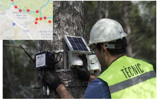
Sensory network for the control and motorisation of natural spaces.
